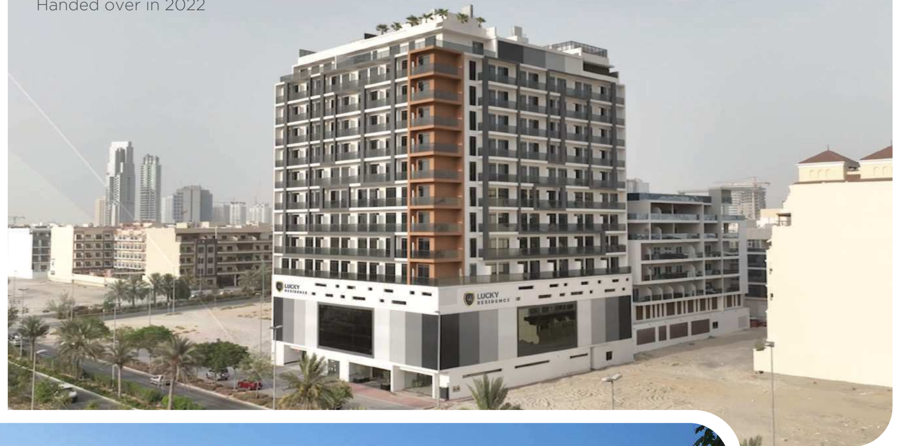
Lucky Residence Handed over in 2022
