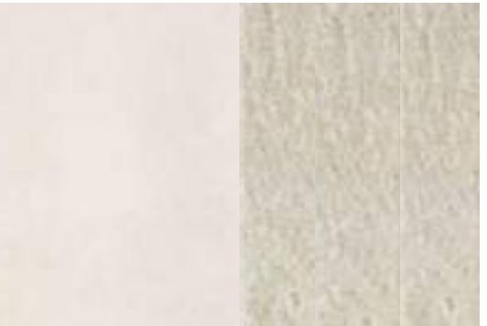
POWDER ROOM WALL AND FLOORING
