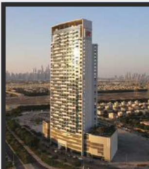
Al Jawahara Tower JVT, Dubai
