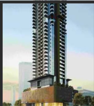
Seslia Tower JVT, Dubai
