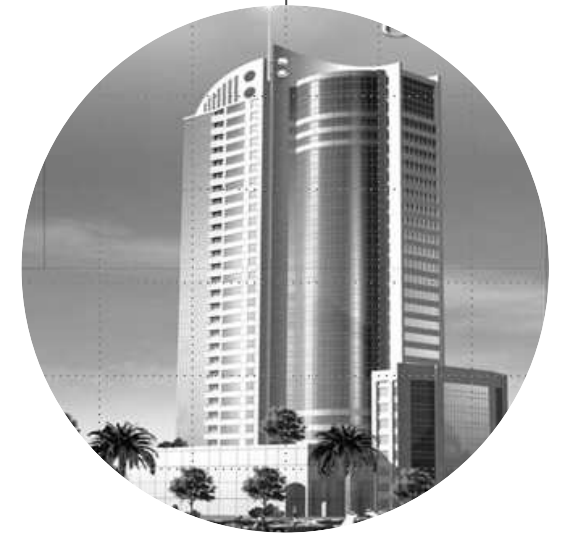
ONTARIO TOWER BUSINESS BAY
